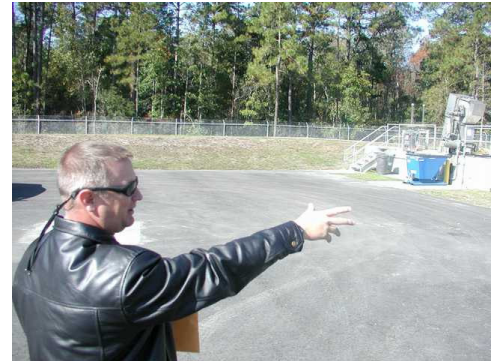
Keith Causeway, project manager with P.C. Simonton & Assoc., Inc., discusses how the plant works.
